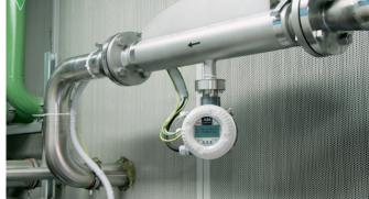
CoriolisMaster Hygienic flowmeter: mass flow measurement for hygienic applications
