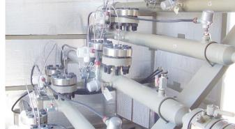
Wedge meters: extremely robust flowmeters for difficult applications Wedge meters are bi-directional and are particularly suitable for fluids which have a high solids content, are erosive/abrasive or have a high viscosity.
