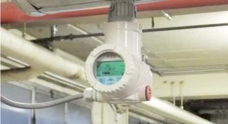
Vortex/Swirl measurement for extremely dynamic flow measurement with high accuracy
